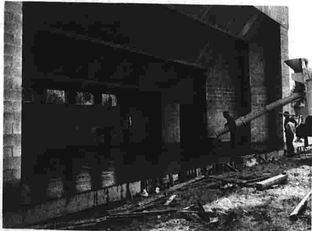
Band shell floor poured
